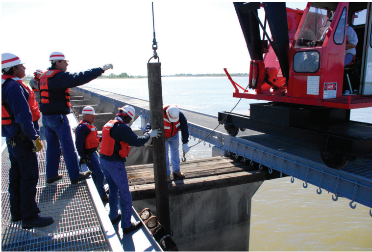
In opening the spillway, each timber is individually lifted and placed atop the structure.
