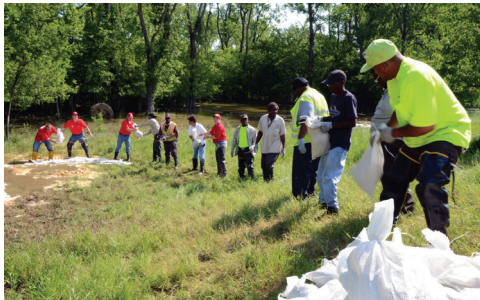
Workers place sandbags near a developing sand boil during the high water event of 2011.
