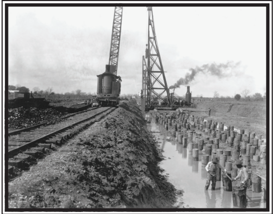
Thousands of wooden pilings were driven to provide a reliable foundation for the spillway structure.
